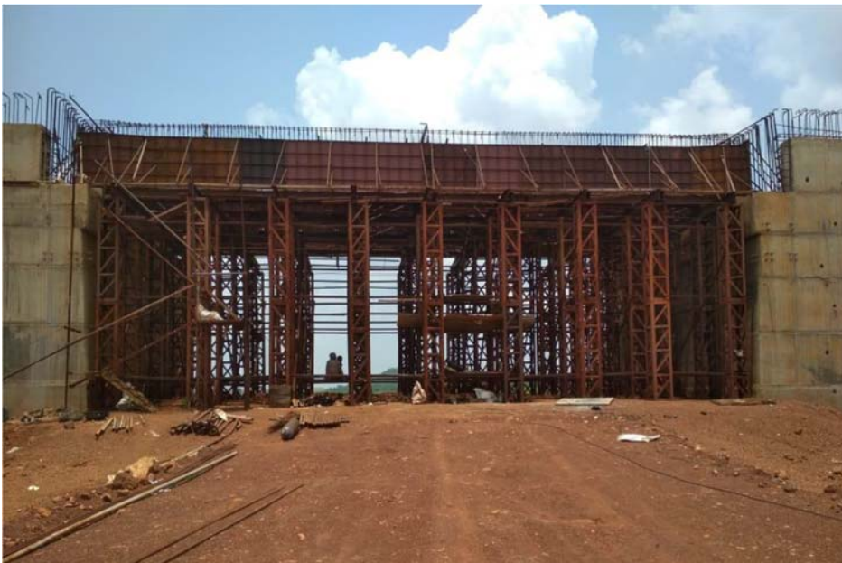
BR. NO.171 SHUTTERING & SUPPORTING WORK
