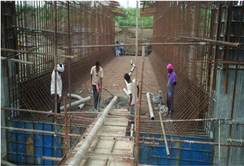
BR. NO.7: RCC BOX BARREL RAFT CONCRETEING
