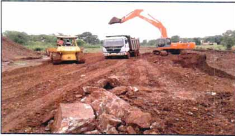
Earth Work in formation between Baliapala (Y Junction) Tomka end.
