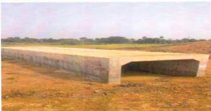
Completed RCC Box near Kamakshyanagar
