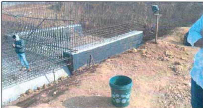
RCC Box Sub Structure work in progress
